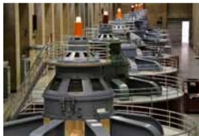
the generator. The giant magnets rotate past copper coils, creating electricity. After the generators produce electricity, it is transferred to an electrical power substation and then transmitted to your home. (June issue of *Alabama Living*, pgs. 6-7).
