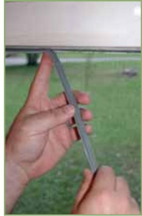
4. Firmly press the adhesive side of the foam weather-stripping to the bottom of the sash.
