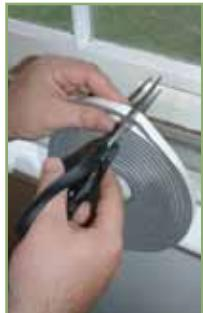
3. With the scissors, cut the foam weather-stripping to the same length as the window sash.
