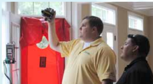
Blankenship conducts an energy efficiency audit on a home, with equipment such as an infrared camera and a blower door.
