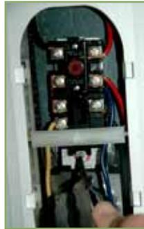
2. Check the temperature setting on the tank. The top element should be set at 120 degrees and the bottom element at 130 degrees for peak efficiency.
