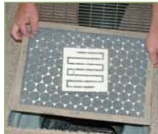
1. Locate your air filter(s). Inspect for debris, dust, hair, etc.
