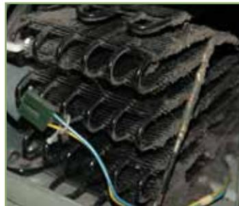
4. Inspect coils for accumulated dirt, dust and grime.
