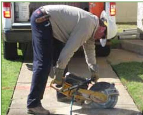
*CAEC Lineman cuts a sidewalk in preparation of underground line installation.*
