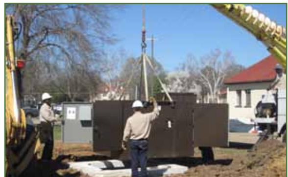
*CAEC Linemen install a primary pad-mounted 600 amp switchgear at Maxwell Air Force Base.*
