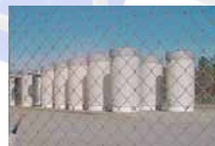
Dry storage photo courtesy of Surry
