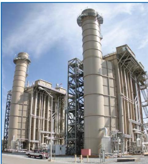
**The boilers for this combined-cycle natural gas plant are surrounded by a system of pipes and tubes and the exhaust towers.**
