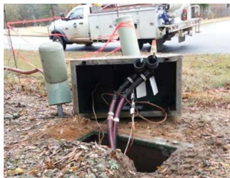
**This damaged underground transformer cabinet created a potentially dangerous situation.**
