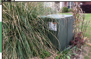
Although plenty of space is left in front of the transformer, overgrown vegetation on the other three sides can cause problems.
