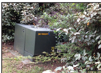
Although plenty of space is left in front of the transformer, overgrown vegetation on the other three sides can cause problems.
